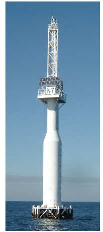
K tower in the Gulf of Mexico.
